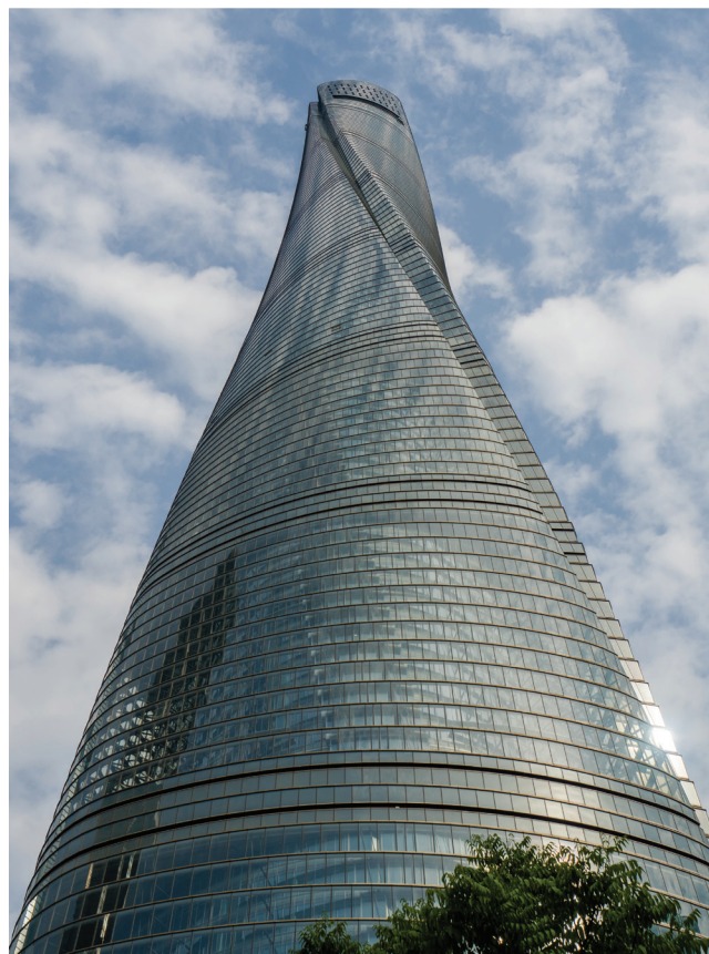
Figure 1: The twisted structure of Shanghai Tower
